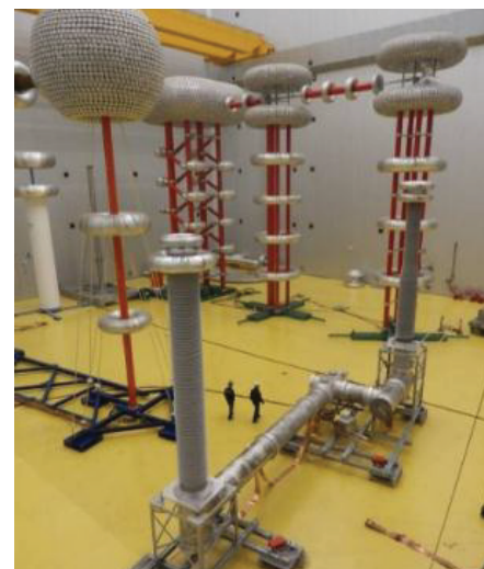
Voltage withstand and bus-charging current switching tests
