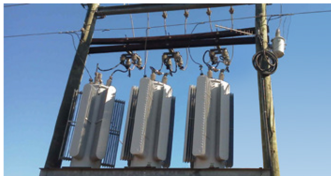
GE Vernova's Pole Mount Voltage Regulator (VR-PM) installed on a platform in a distribution network
