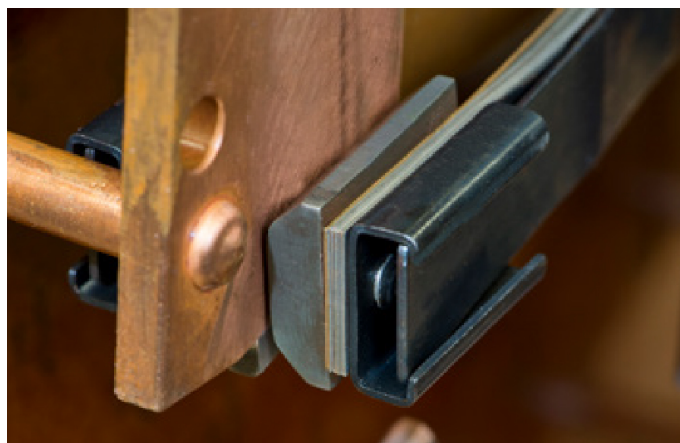
Moving switch contacts
