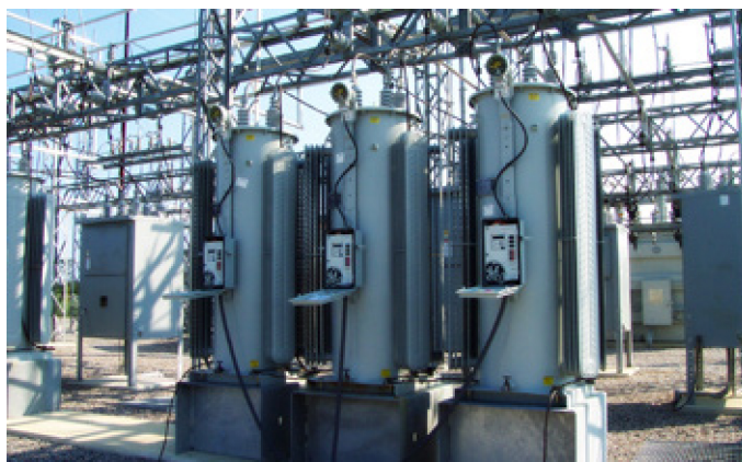
GE Vernova's Substation Voltage Regulator (VR-SS) installed on a distribution network
