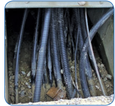
Extensive amounts of copper cables need to be distributed from each switchyard apparatus back to the control house
