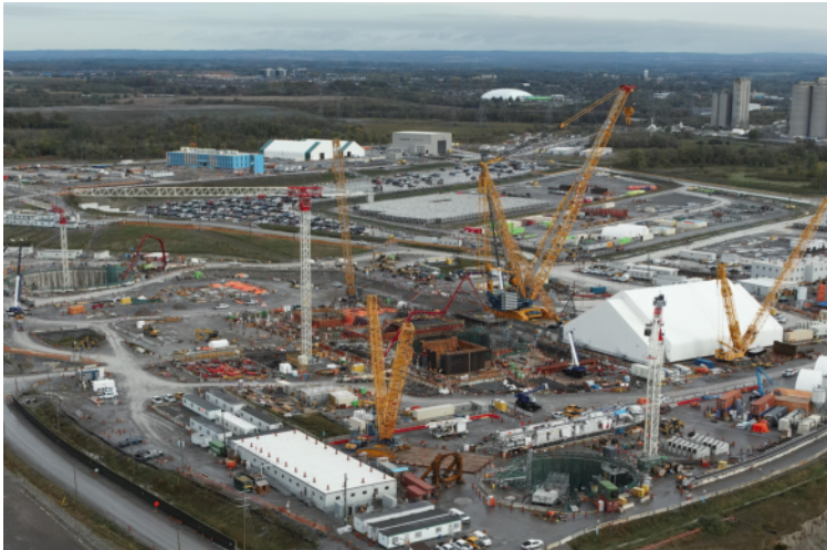
Construction on the GE Vernova Hitachi BWRX-300 continues to progress at Ontario Power Generation's Darlington site.
