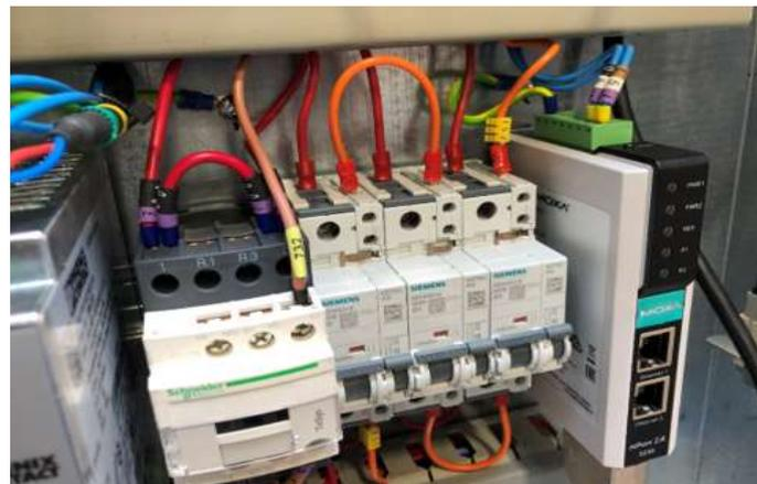
Cooling Kit MCB's installed and wired ready for test
