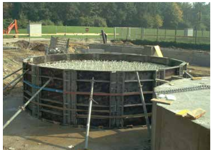
Foundations of the TCR reactors with GRP reinforcement
