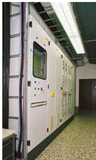
Figure 1: Cubicle blocks with 4x ±1200 kvar water-cooled, modular PRO-X pulse inverters, open and closed-loop control for the 16 modular inverters and one of the four converter transformers with gas-insulated compact switchgear.
