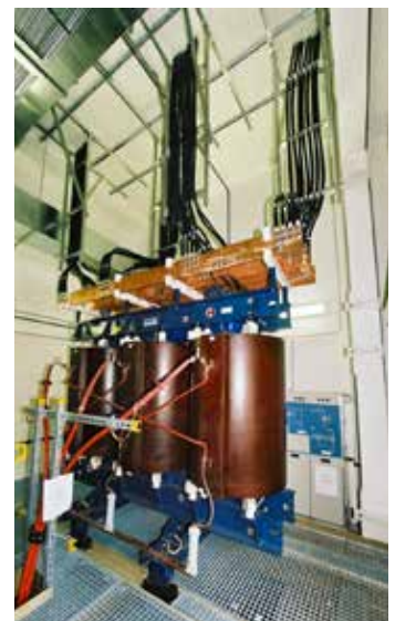
Figure 1: Cubicle blocks with 4x ±1200 kvar water-cooled, modular PRO-X pulse inverters, open and closed-loop control for the 16 modular inverters and one of the four converter transformers with gas-insulated compact switchgear.
