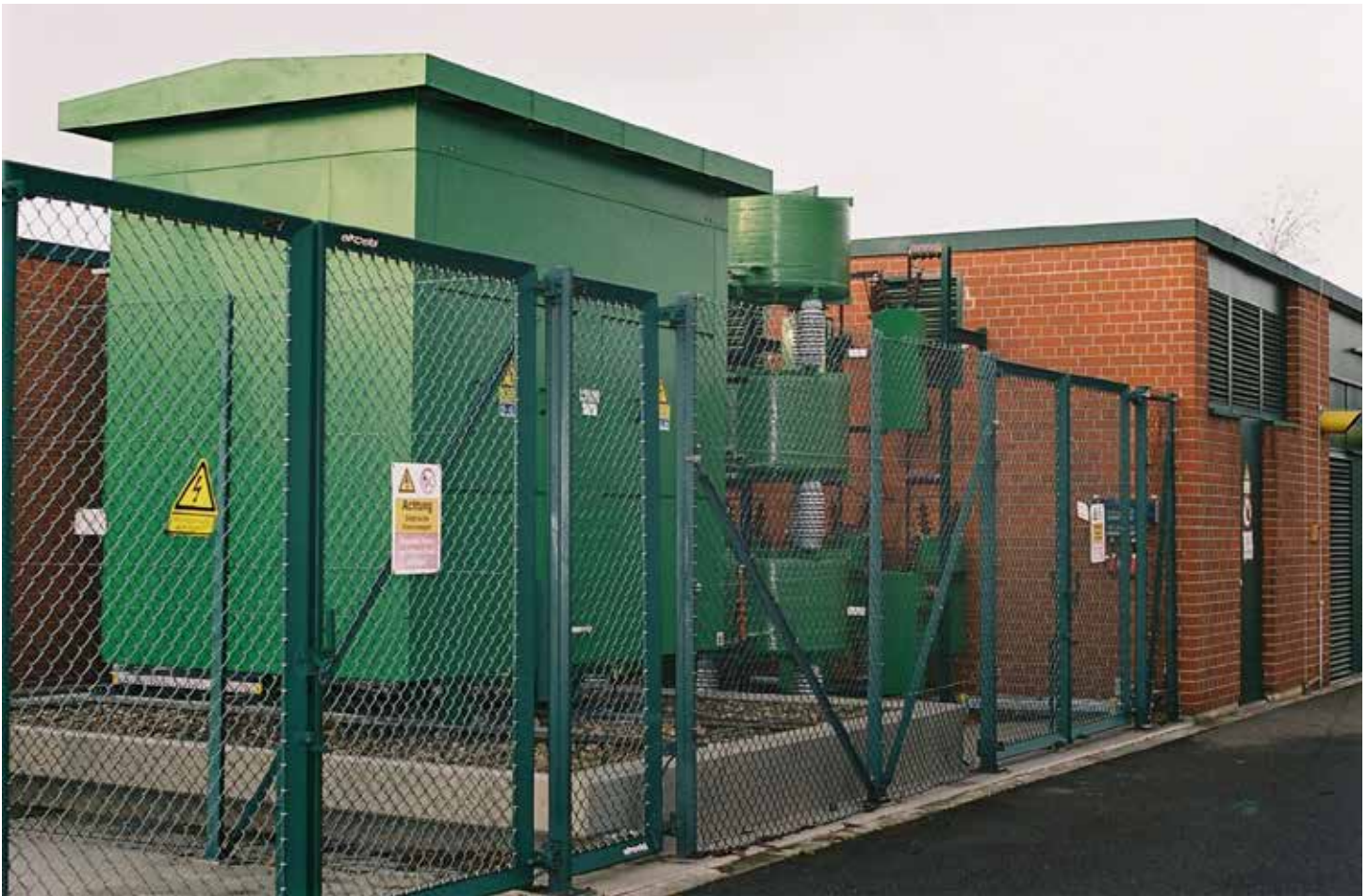
Figure 12: Cast resin transformer in outdoor housing, outdoor harmonic filters
