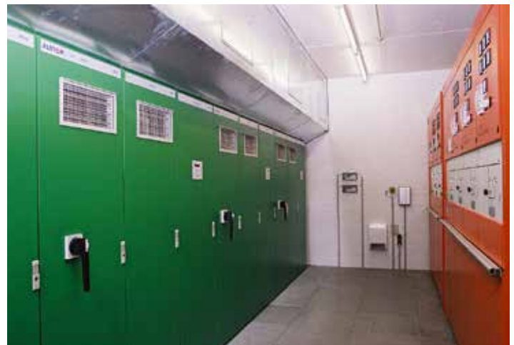
Figure 1: Row of four \pm 812.5 kvar cubicles based on MD2000 pulse inverters installed close to 20 kV switchgear and closed loop control
