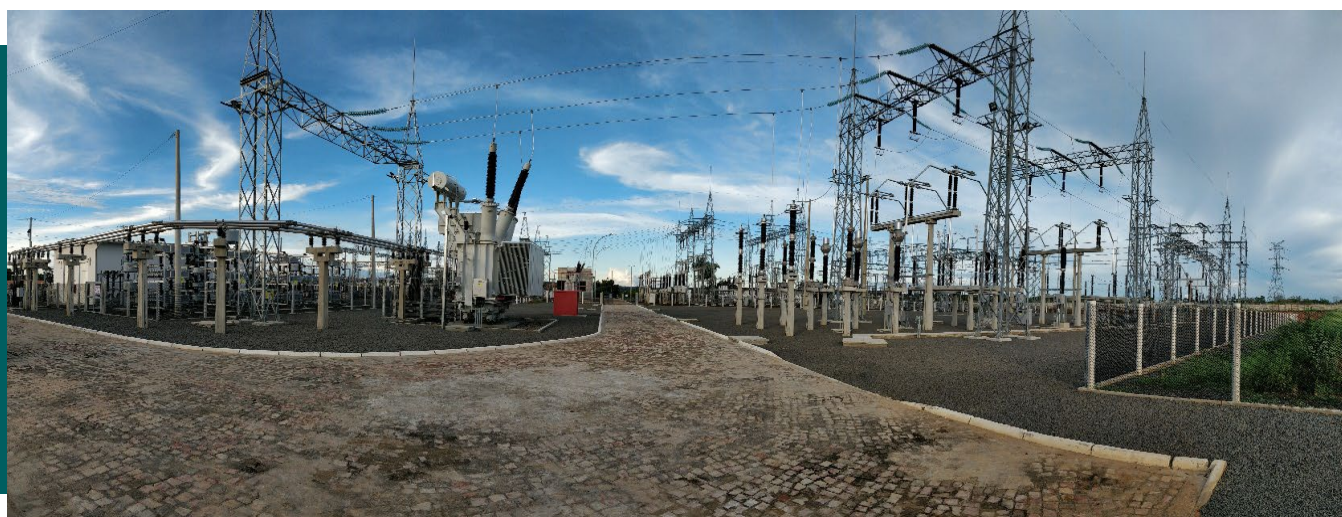
The dynamic compensation system on the left and substation on the right
