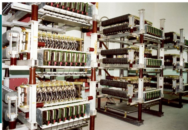
Three-phase frames of thyristor converter
