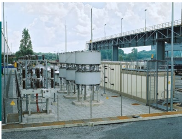
Split reactor coils of the TCR
