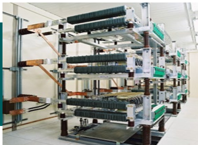
Tree-phase assemblies of the thyristor rectifier in the container
