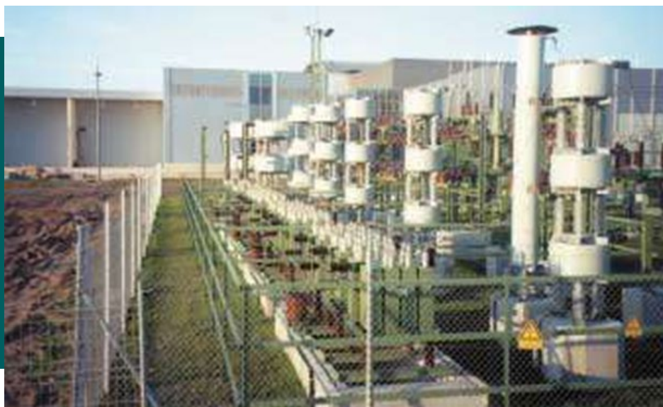
Outdoor area with reactor and five filter circuits
