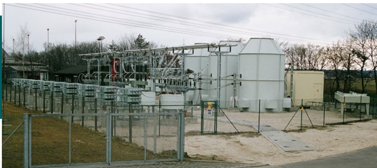
Outdoor installation with filter circuits and sound-insulated TCR reactor coils
