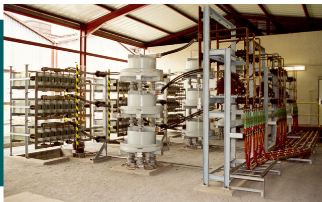
Filter circuits in a tower structure
