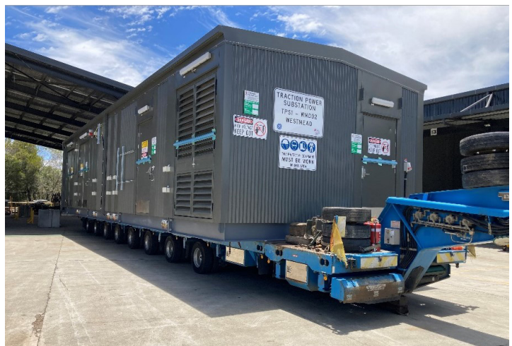
Off-site traction power substation construction
