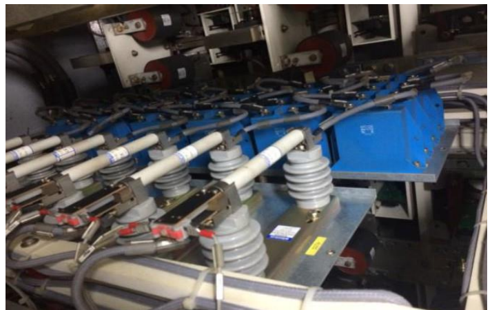
Varistor and fuses of SD7 drives
