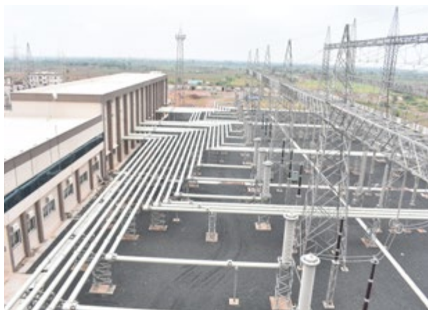
400/220kV GIS for GETCO at Shapar
