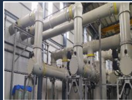
Six bays of 220 kV GIS with 1200 meters Gas Insulated Busbar for Sterlite's project for PGCIL at Vadodara Gujarat
