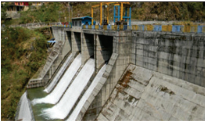
2 x 55 MW Chuzachen Hydro Electric Project successfully commissioned by Alstom
