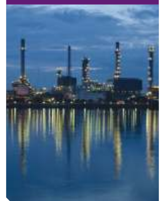
Electrical Automation Solutions for Refineries
