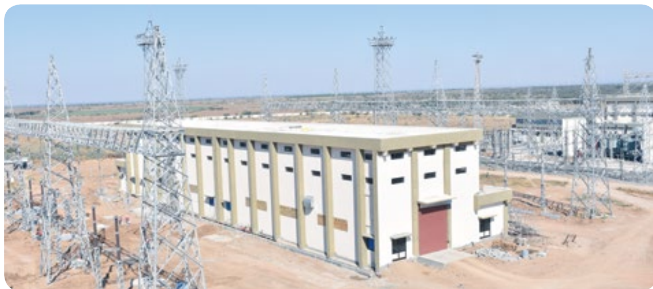
400 kV Gas Insulated Substation for Gujarat Energy Transmission Corporation Limited (GETCO) at Bhachunda, Gujarat
