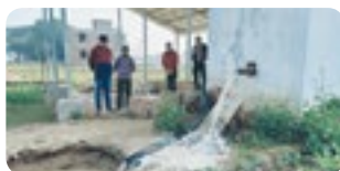
Installation of solar pump at Naini
