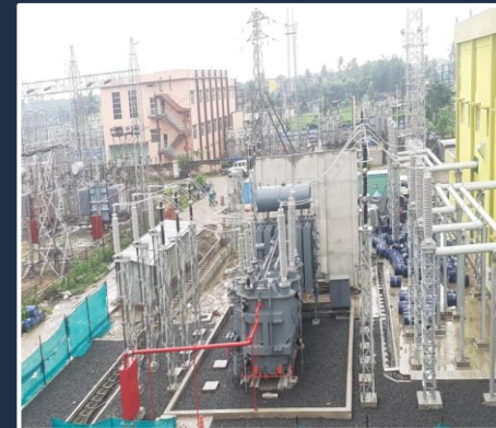
7x220 kV GIS bays, 1x160 MVA ATR, 1 X132 kV AIS Bay charged for DVC at Burdwan
