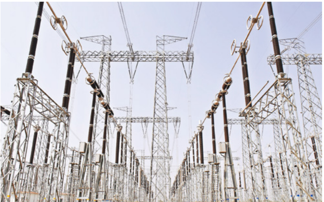
▲ Execution excellence in turnkey solutions
