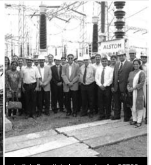
India's first digital substation for GETCO
