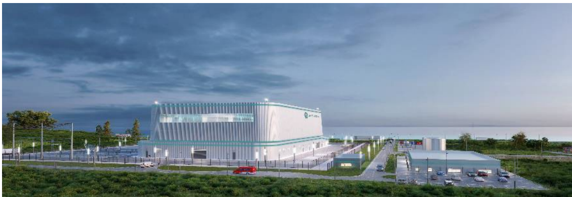
Planned BWRX-300 by Ontario Power Generation at Darlington
