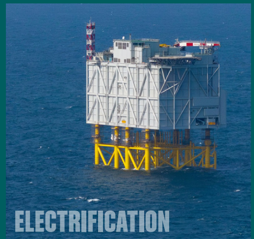
Installation of GE Vernova’s HVDC offshore converter platform for RWE’s Sofia Wind Farm in United Kingdom waters (Credit: RWE)
