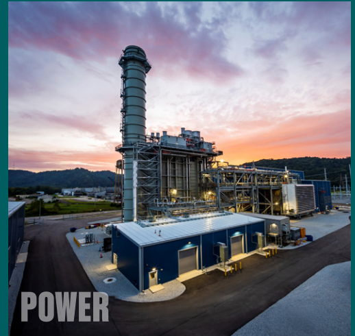
GE Vernova’s 7HA.02-powered Long Ridge Energy Terminal in Ohio, the first hydrogen-burning power plant in the U.S.
