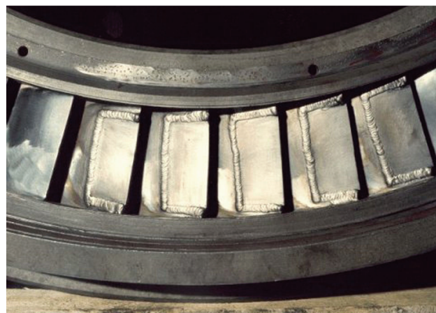
Diaphragm insert repair prior to dressing
